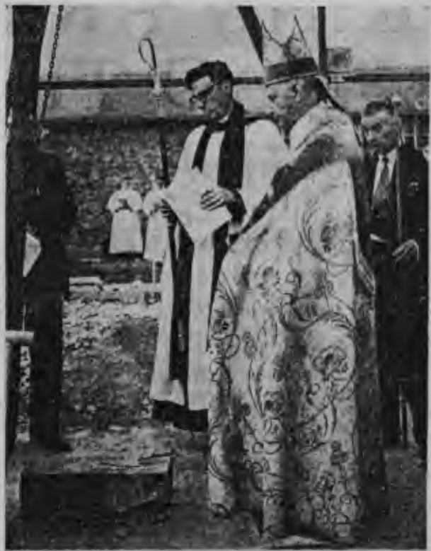
The Bishop of Lincoln, Rt. Rev. Kenneth Riches, lays the foundation stone of the Church of St. John the Baptist, on Ermine Estate, Lincoln. The stone, which is taken from Lincoln Cathedral, is unusually placed, being in the centre of the church.
